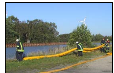
Placing the barrier into the water
