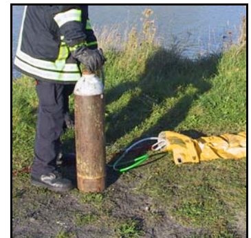
Filling the barrier from a compressed-air cylinder
